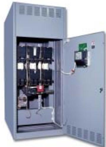
**Fig. 6:** ASCO Power Transfer Switch rated 3000 amperes
