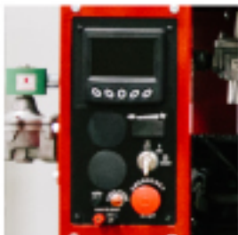
Murphy PV 480 Control Panel / Electronic Throttle and E-Stop
